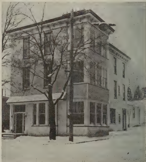
The remodeled building as it now appears, an up-to-date apartment house. The frame side extension, providing a sun-parlor in each story, is new. The old school house, as remodeled, can be seen to the extreme right
